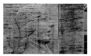
Figure 3. Fragment of the travertine relief of Freedom Monument 2 years after restoration and hydrophobic treatment without any maintenance. Left side of the figure shows the hydrophobic surface, the right side - untreated surface. The untreated surface shows uniform soiling while treated surface has heterogeneous dislocation of soiling in the form of vertical run-off lines.
