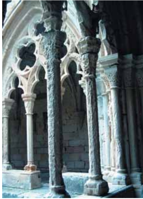
Figure 3: The decay of materials (cloister of the Monastery of Poblet, Spain)
