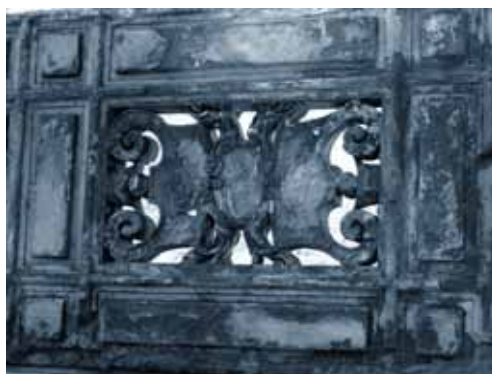
Figure 2: Perfectly conserved areas of the surface of stone and areas from which the fluted layer has broken away
