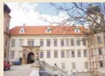
Example of application of lime – metakaoline mortar at two layers (coarse and fine stucco layer). Mníšek pod Brdy Castle, in Central Bohemia, CR.
