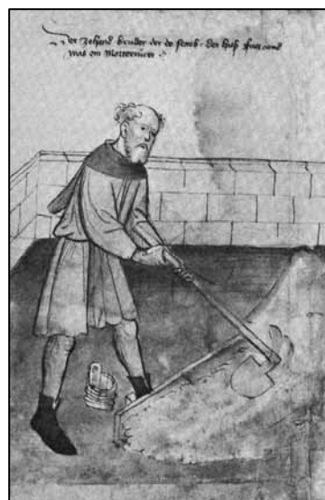
Figure 2: Medieval mortar mixer at work, drawing in town archive of Nürnberg, after 1425
