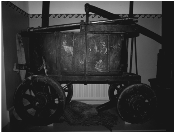
Picture left. Man powered fire pump from 1850's in museum of Pietarsaari. Pump capacity about 80 l/min. Photo R.S.
