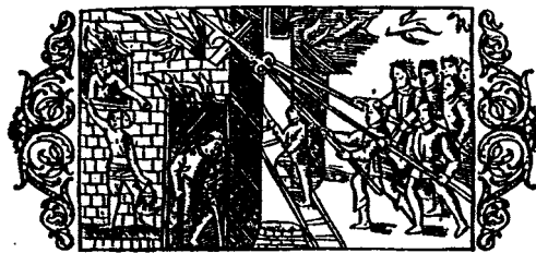
Picture. Fire fighting in 16 th century according to a drawing by Olaus Magnus. Burning particles are being pulled down from the roof by fire hooks. Ladders and water buckets made of leather can be seen as other fire fighting equipment. These methods were used in Northern countries until late 18 th century.
