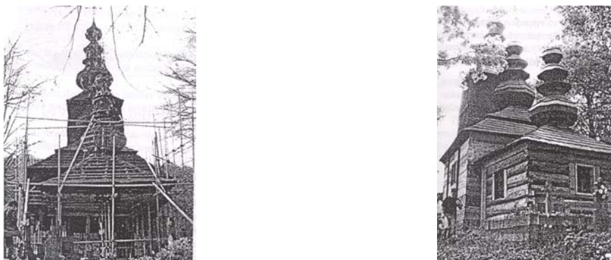
Figure 2: Wooden church in Hunkovce during and after renovation
