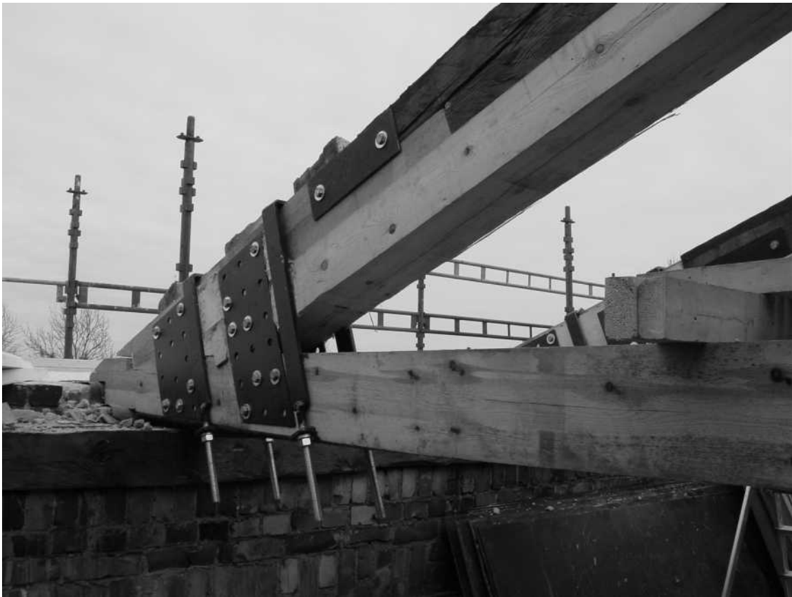
15. Artillery manege, joints has strengthen
